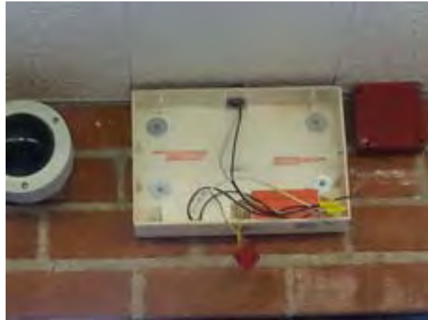
Disabled fire alarm sign with exposed wires
