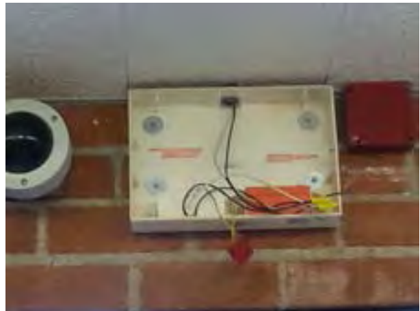
Disabled fire alarm sign with exposed wires
